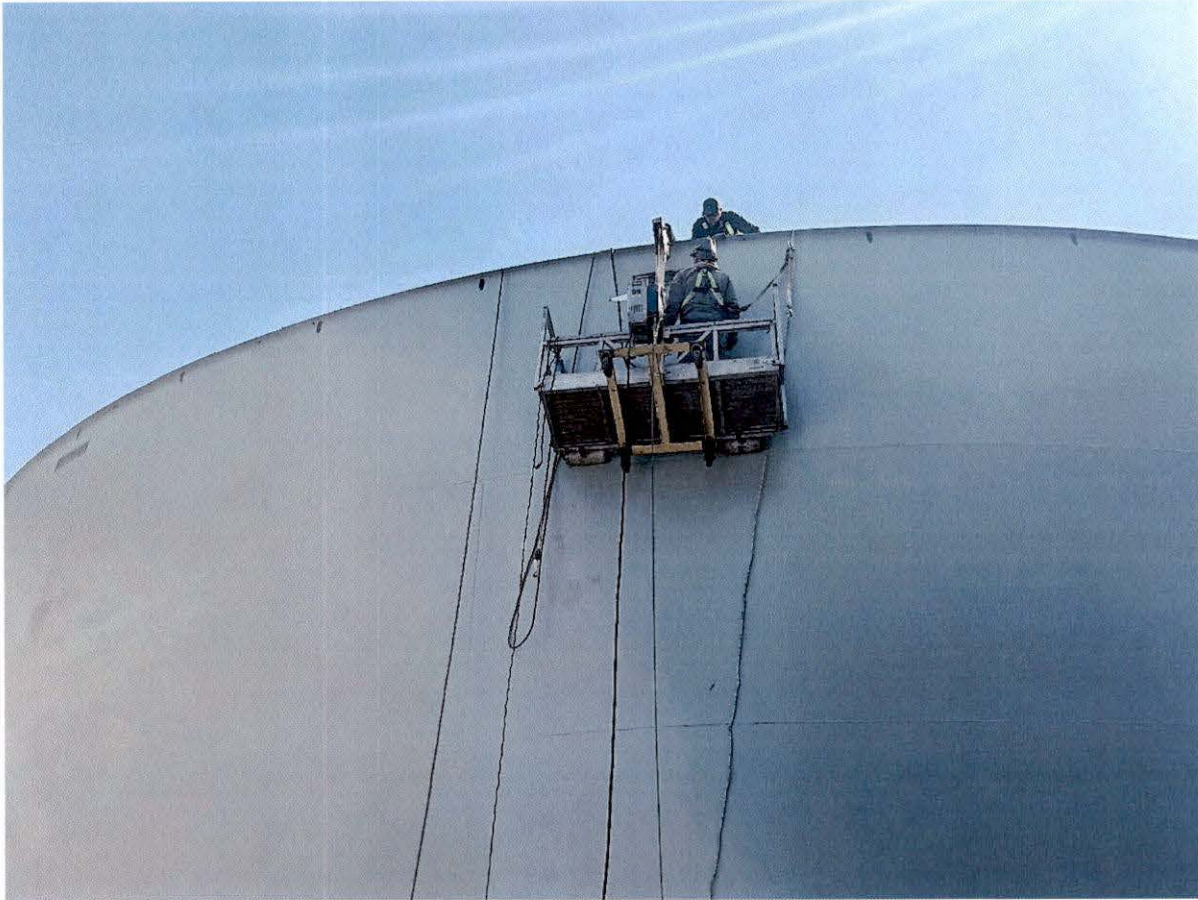
March 3, 2026 – Welding shell vents.
