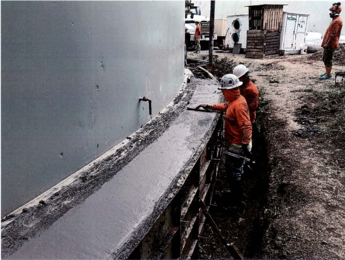
March 30, 2026 – Finishing/troweling the concrete ringwall extension.
