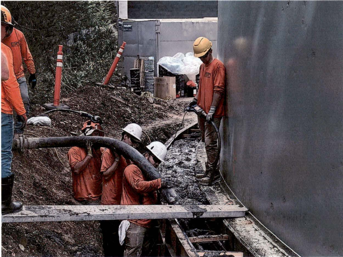
March 30, 2026 – Pouring concrete ringwall extension.
