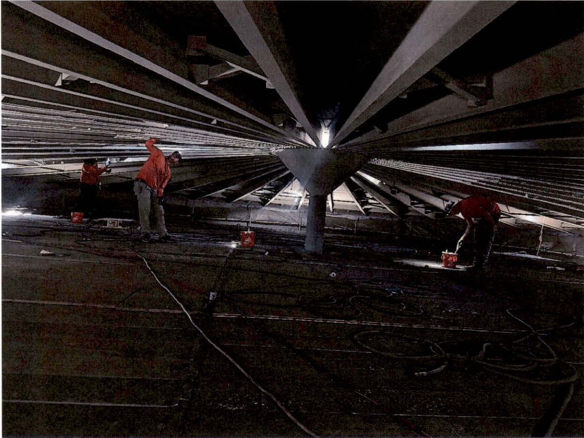
March 24, 2026 – Applying the 1 st coat on the interior roof.
