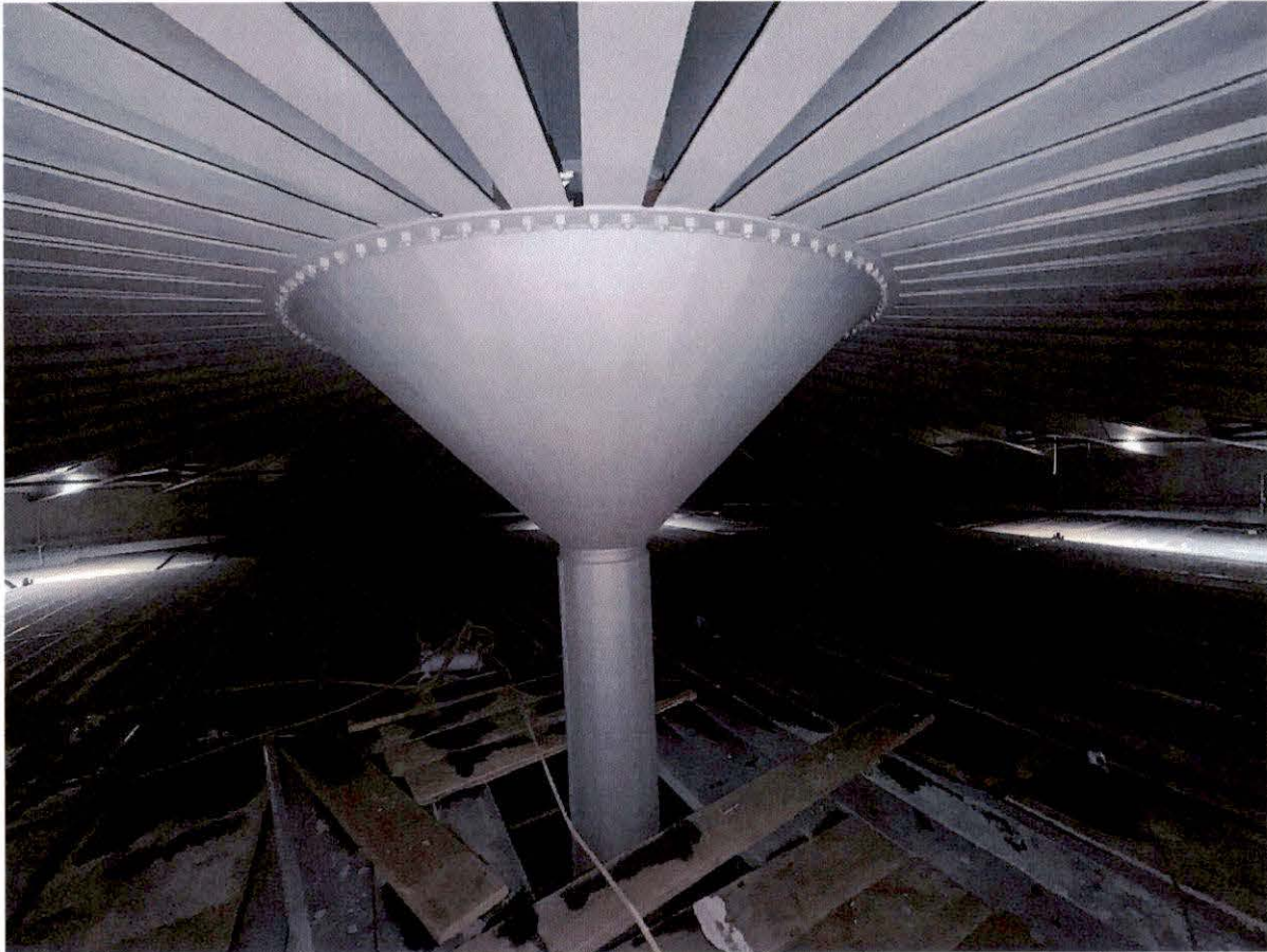
March 18, 2026 – View of sandblasted center column and rafters.
